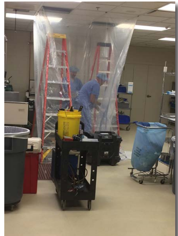
Emergency repair of a deionized water line on the dirty side of the sterile processing department (SPD). A barrier was created with HEPA filtration to contain everything possible.
