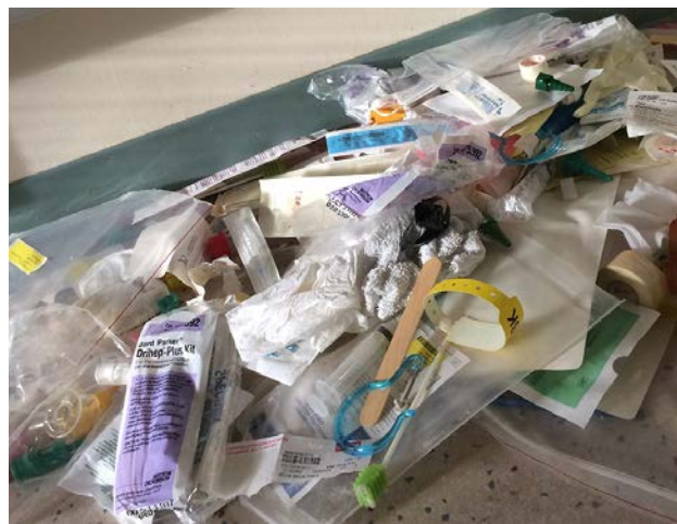
While working on an oxygen outlet, the head wall needed to be removed and this is what was found. Hospital staff was notified immediately, some of it dated back to 1978.
