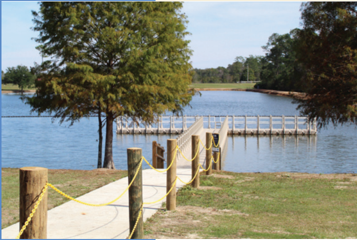
The completed fishing pier
