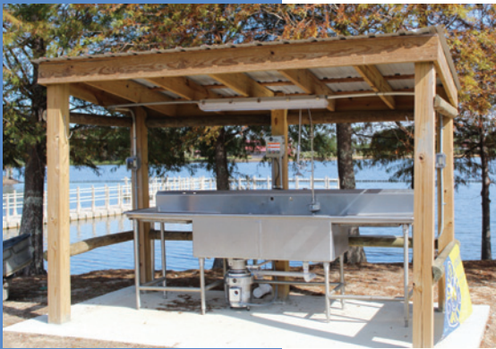
The completed fish-cleaning station
