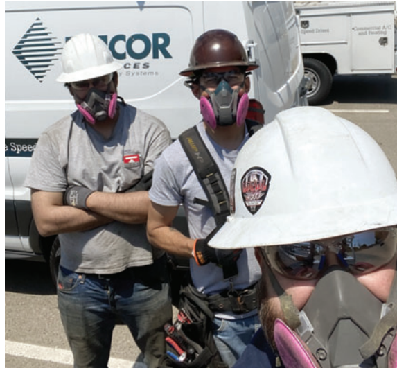
Members are shown on a job for the County of Fresno. Pictured from left are apprentice refrigeration fitter Ihab Kharda, apprentice refrigeration fitter Carlos Rendon, and journeyman refrigeration fitter Ray Valladares.
