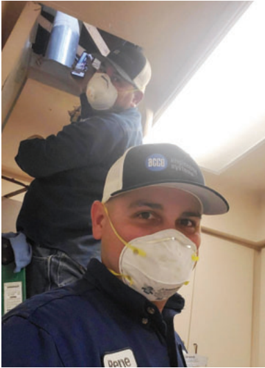
UA Brothers Rene Alvarado and Catarino Jimenez are pictured on a service call to repair a domestic hot water leak at the Reedley Palm Village Retirement Home.
