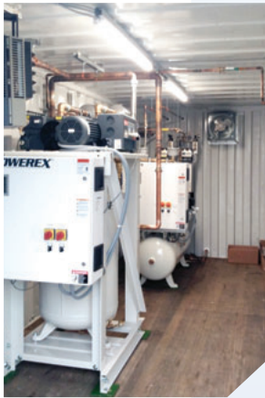
W.E. Bowers portable mechanical room inside a sea can
